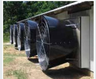
Flush mount design allows retrofit over wall openings from 57.5" to 63"
